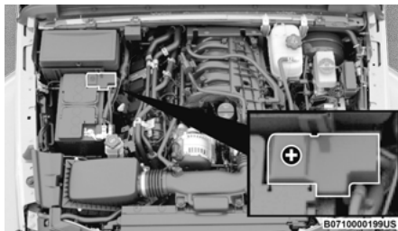
Positive (+) Battery Post – Gas Engine
